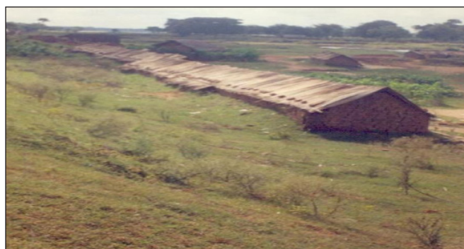
Plate 14: Temporary sheds near brick-kilns
